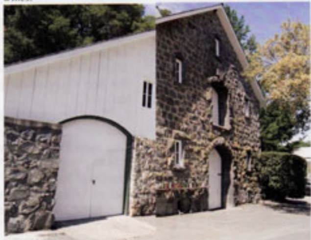
The old wood-floored wine cellar, built in 1898, still holds barrels and fermentation tanks for Heitz wines.
